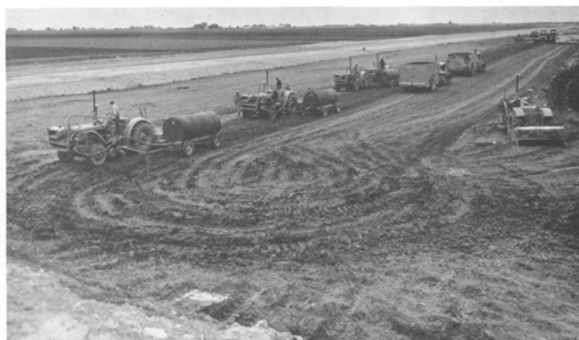
Figure 16. Embankment construction, loop 1, using rotary speed mixers to process and adjust moisture content of soil.
