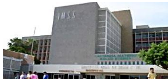
Figura 6. 1 Hospital General IMSS, Querétaro
